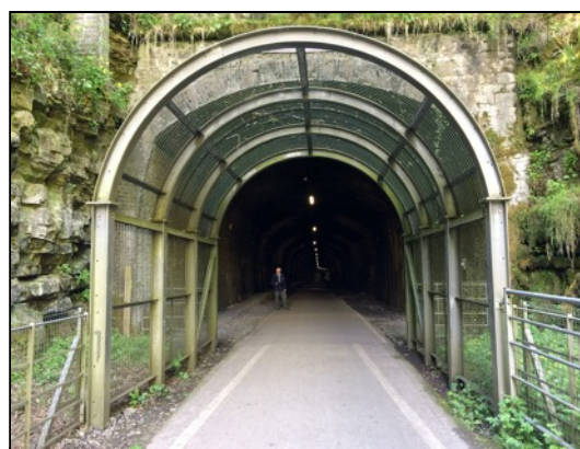
The protective steel cage
