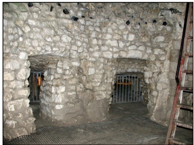
Figure 2 Note the hard black flint in the wall
