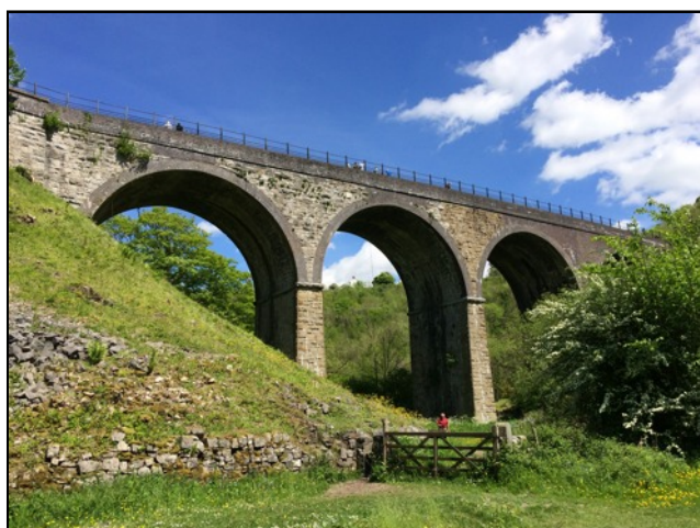
The Headstone viaduct from below
