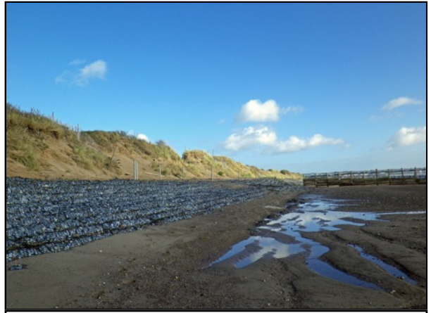
Fig 2 Dunes, gabions and foreshore of Dawlish Warren.
