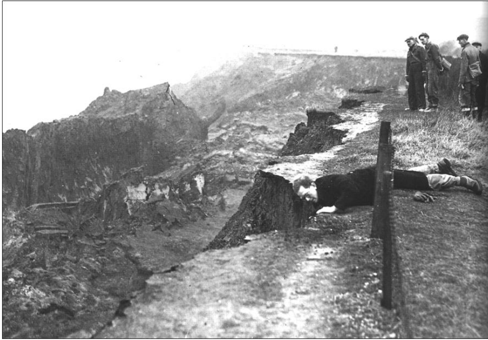
Figure 3 – Gas Engineer looking for a broken main caused by this major landslide at the Miramar Hotel in Beltinge
