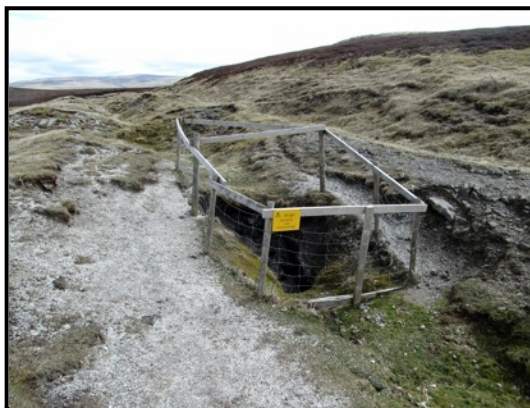
Fig 6 Disused Lead Mine Shaft
