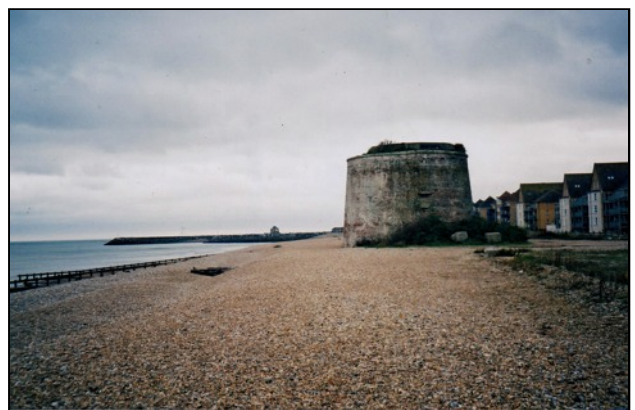
Fig 1 Martello Tower No.64
